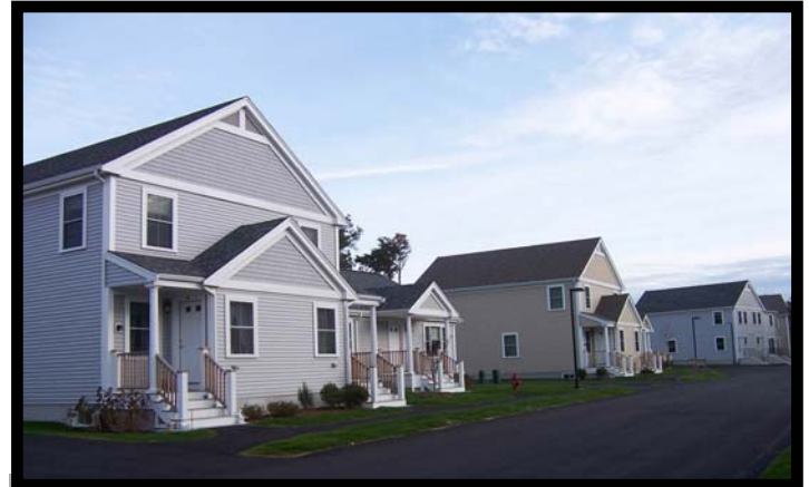
Chatham used $300,000 in CPA funds to support the construction of 47 affordable rental units on housing authority land.
