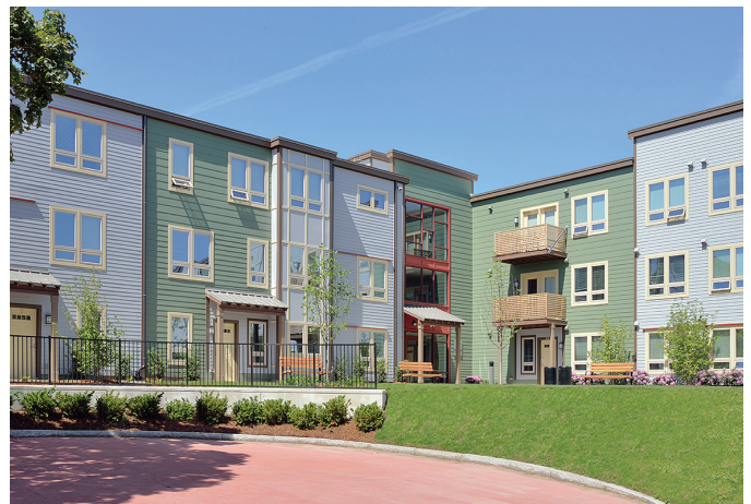
St. Polycarp Village Phase III, Somerville.
