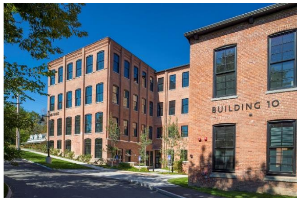
Cable Mills, Williamstown
